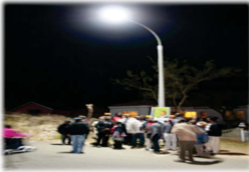
Retrofitted street lights in Kocksoord and Merafon.
